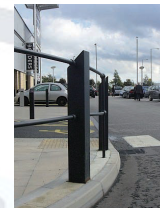
Bollard combined with hand rail
